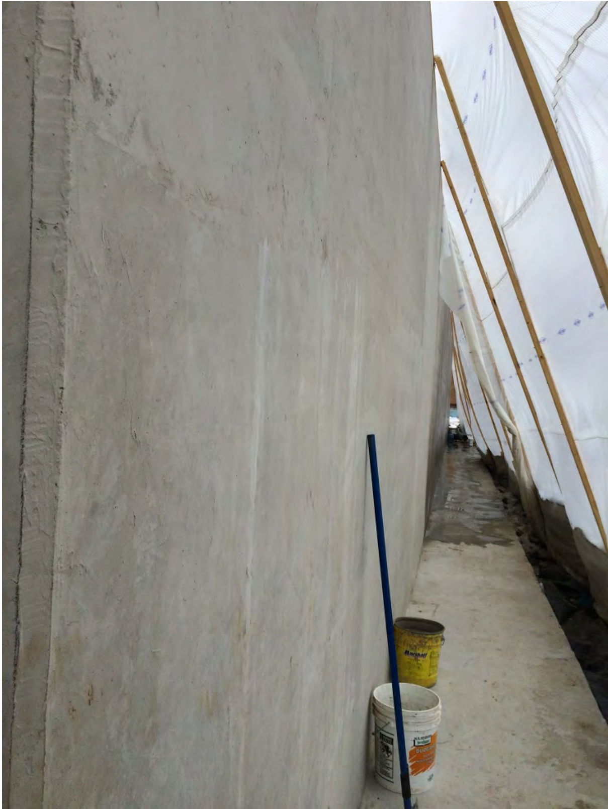
Foundation wall ready for Waterproofing install.
