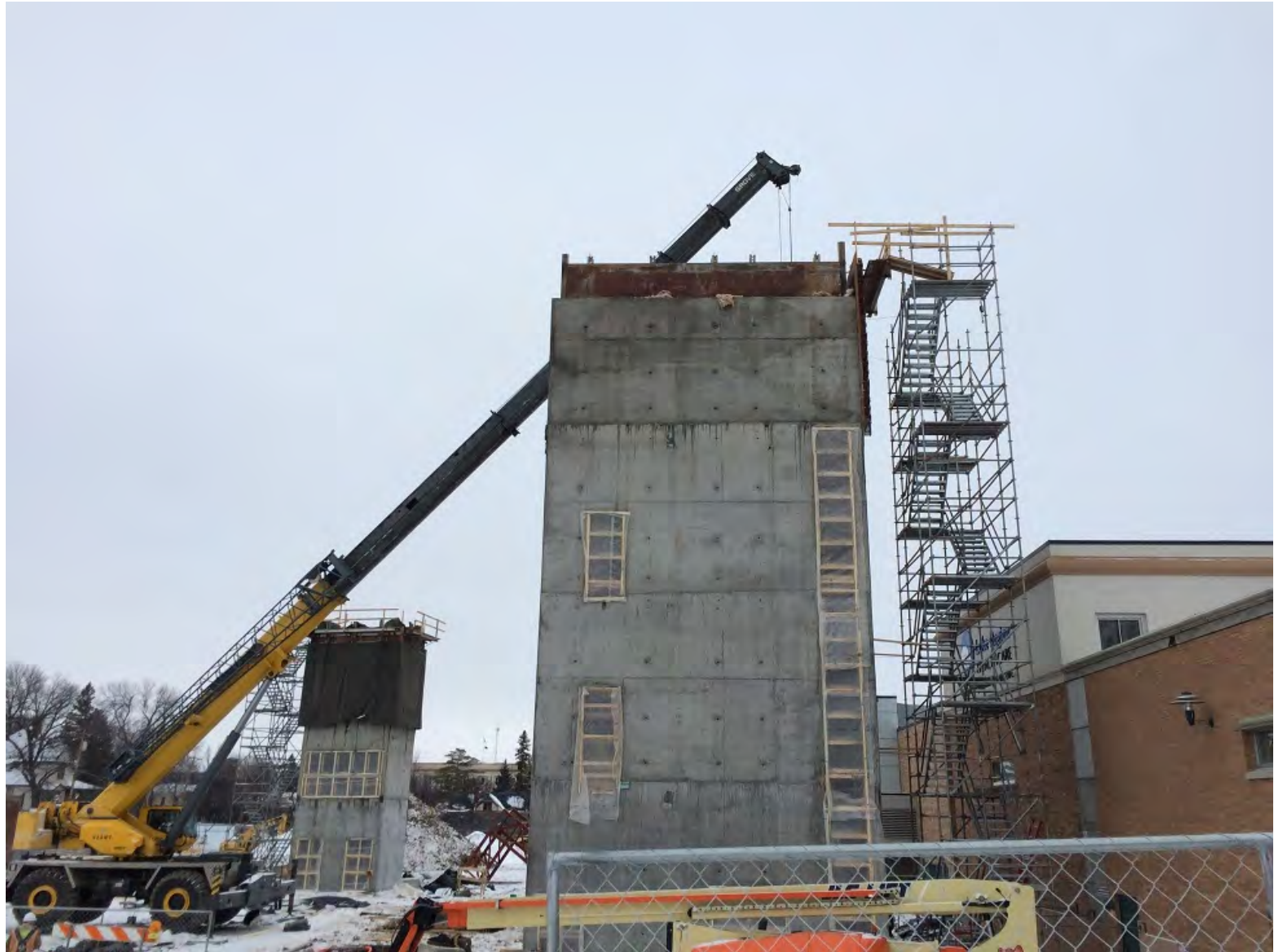
4 th and final level of Stair B Poured.
