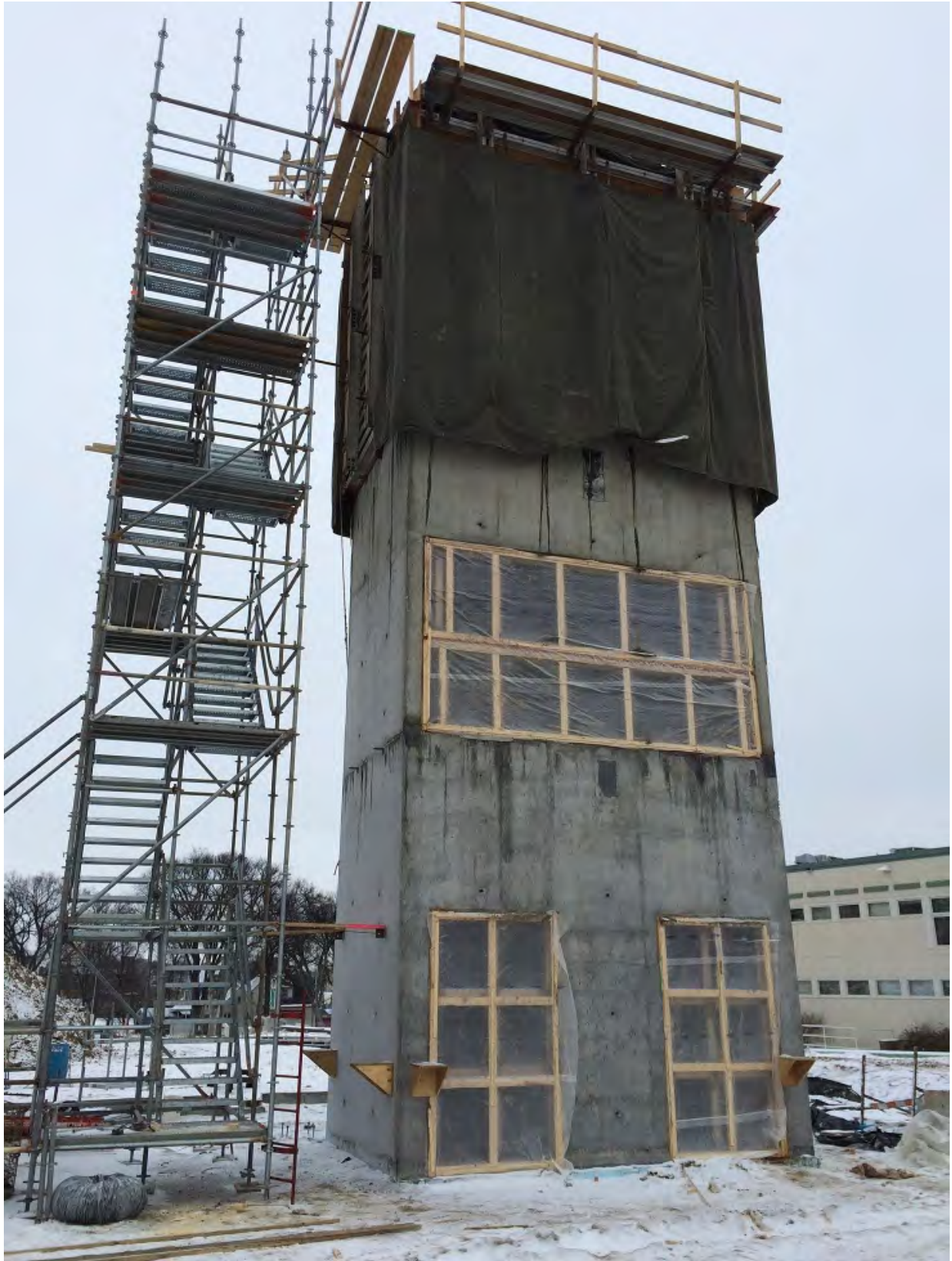
Poured 3rd level of double elevator core wall.
