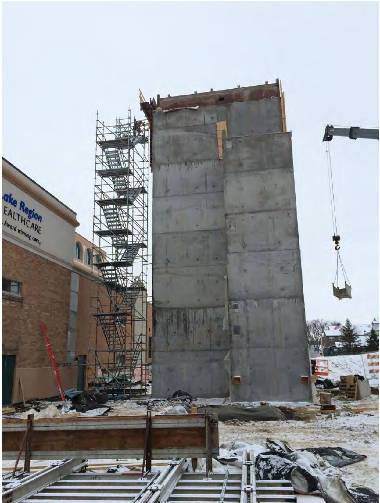
Stripping off forms on Stair B.
